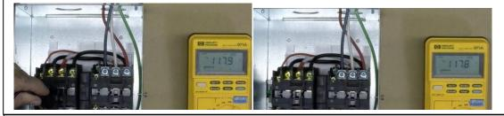
6. The center of the Generator contactor should be in the down position, if it is not the switch is defective.
