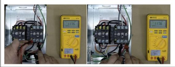
3. With the shore power on and the main breaker off. The center of the shore side contactor should be in the down position, if it is not the switch is defective.
