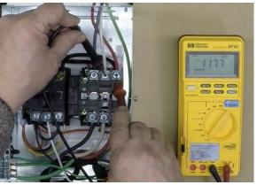
4. Generator side. Turn on the generator. In 20-30 seconds the green light on the side of the contactor will illuminate and the generator contactor will go down, (engage). The shore side contactor will release as this is happening.
