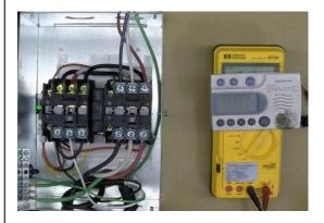
5. To check the output from the generator . (Input to the contactor.)
