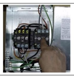
2. With the shore power on and the main breaker off. Measure between the neutral and Hot 1, then the Neutral and Hot 2 Where the shore cord connects to the contactor.
